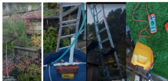
Figure 7. Header, Ram pump, Delivery, Micro turbine voltage measurement
